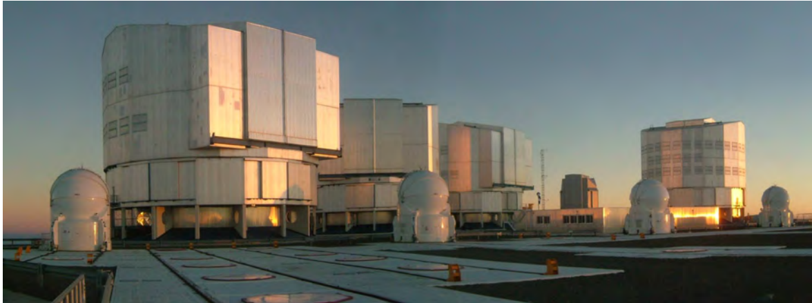
Figure 2.6: Photo from the VLTI platform. On the image, the four unit telescopes (UT1, UT2, UT3 and UT4 from left to right) and the four auxiliary telescopes can be seen. Between UT3 and UT4, the VLT survey telescope (VST) towers behind the interferometric laboratory. The rails in the foreground are used to move the auxiliary telescopes; the octagonal covers mark the position of the VLTI stations.
